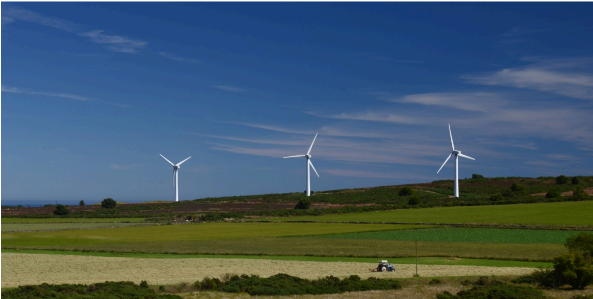
Figure 13.11. Wind farm in Kempstone Hill, Scotland.
