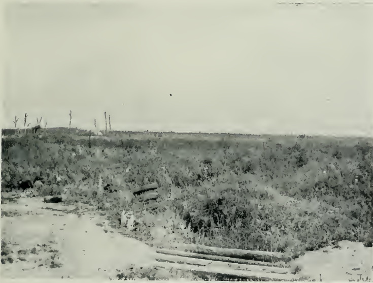
The trenches at Potijze, looking towards Verlorenhoek.
