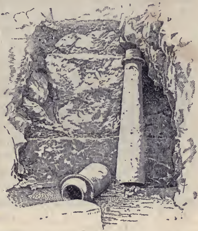
FIG. 142. TILE DRAINPIPES FROM THE CRETAN PALACE OF CNOSSUS
