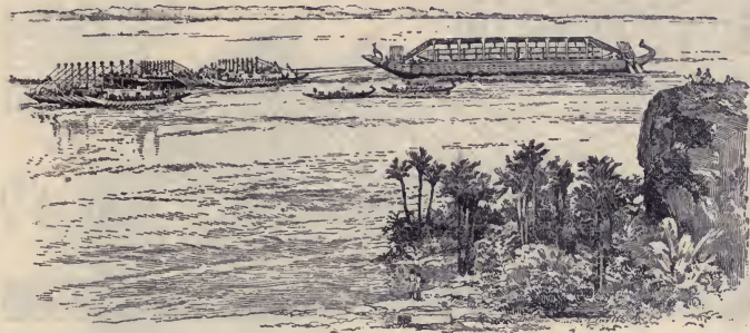
FIG. 61. TRANSPORTATION OF QUEEN HATSHEPSUT'S 350-TON OBELISKS DOWN THE NILE (FIFTEENTH CENTURY B.C.)
