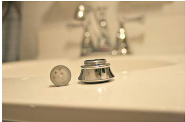
Figure 4.11: Faucet aerator illustration.
