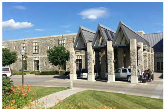
Figure 16.8: The Inn at Virginia Tech, managed by Benchmark Hospitality.
